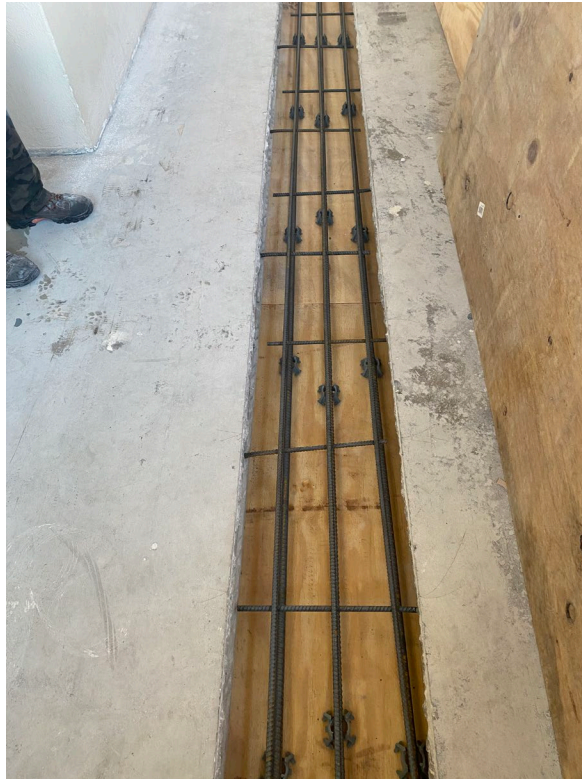
Picture 1: 7 th floor North walkway full depth repair
